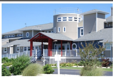
Energy Audit and Systems Design Children's Beach House
