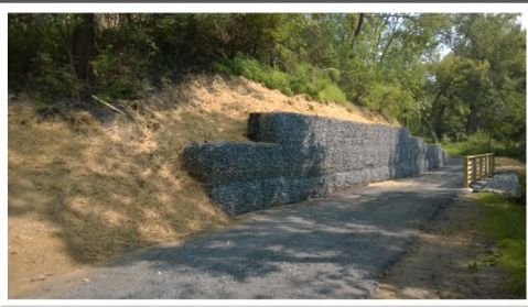
Ironton Rail: Rails to Trails North Whitehall Township
