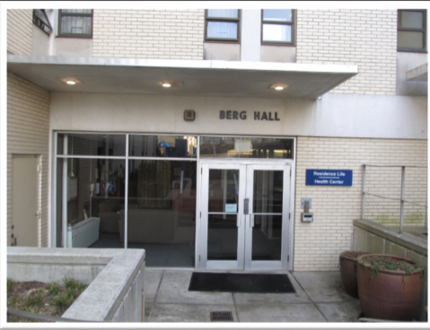
Dormitory HVAC Conversion Marymount University
